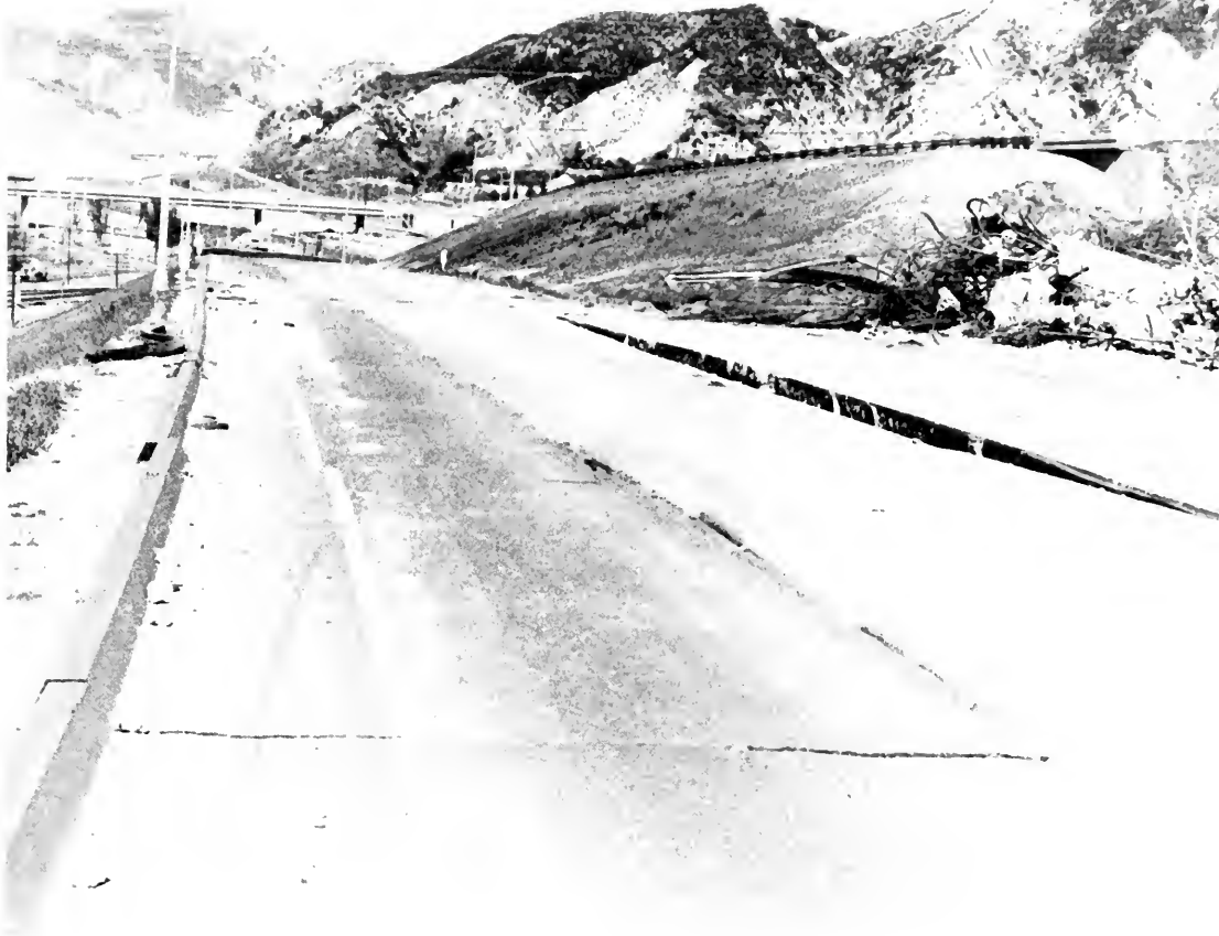
Photo 5. Vertical and horizontal offsets in concrete pavement slabs caused by shear failure in fill material.
